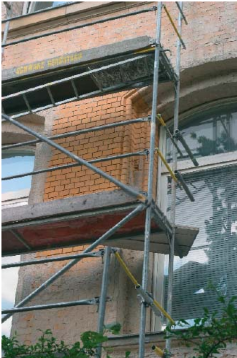
sample area of the restored façade
