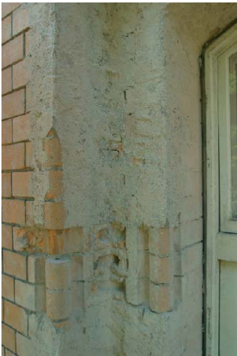
actual condition of the façade
