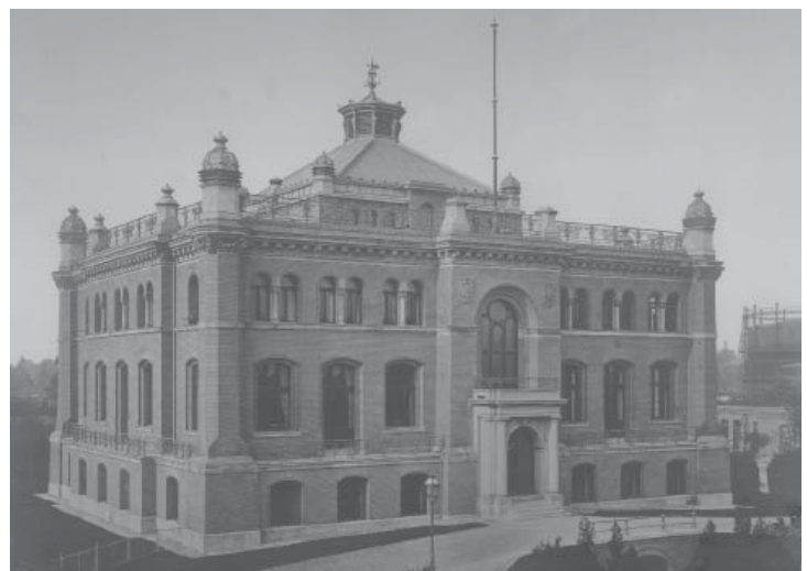
historical view of the building
